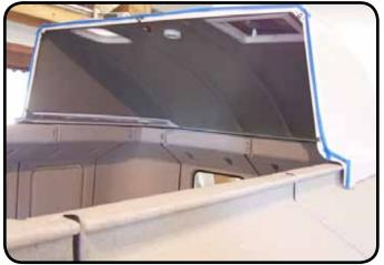
Place a primary roof section so the flat portion of the roof lip that has the foam seal rests on top of the panels. Scoot the roof as far as it will go toward the center of the shelter.
