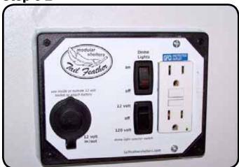
Once 120 volt power is provided, press the reset button on the outlet all the way in until it clicks and the small green light illuminates. Use the bottom switch to choose between power sources for the lights. The upper switch turns on the lights.
