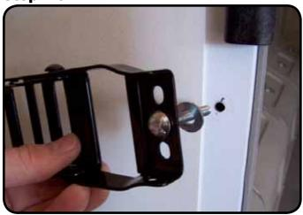
Install the assembly/safety strap buckle to the left side of the doorframe using the bolt, spacer and wing nut supplied with the buckle. The spacer provides room for the strap to be threaded.
