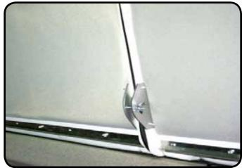
Use the 1/4" screws and wing nuts to join the roof flanges. **IMPORTANT:** Do not over tighten! Watch the gap where the roof flange seals meet and only tighten the screws until no light shows through the gap.
