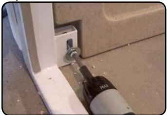
Use a screw and washer to attach the bottom left hand corner of the door frame to the end panel.
