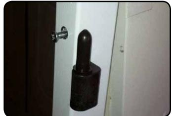
Tighten the four screws to draw the wing up against the door post. Make sure that the door post is fully seated in the wing channel, but do not over tighten.
