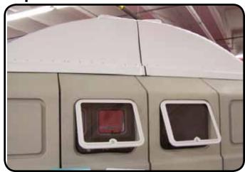
Place the other primary roof section on the opposing end of the camper/shelter. Slide both roof sections together. (See next step for longer roofs)
