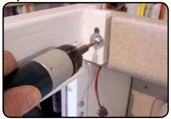
Attach the upper left hand door frame tab to the end panel with a screw and washer.
