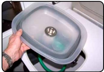
Place the collapsible sink in the counter top and twist the hose over the hose bib located on the door frame. Push down on the bottom of the sink to pop it into it uncollapsed configuration.
