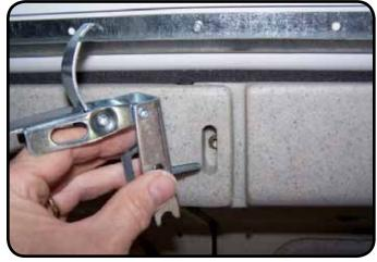
Roof hold-down clamps should be placed near the four corners of the roof. On longer roofs extra clamps can be placed near the center. Remove the panel screw and use the screw without a washer to attach the roof clamp.
