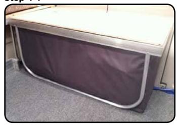
Test the bench to make sure it is tightened up to the wall. Recheck straps. Some play is normal.
