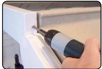
Looking at the door frame from outside the camper, insert the anchor screw in the upper right hand corner. Make sure the screw lines up with the slot in the side panel tab.
