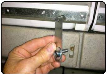
Install the roof safety clip under the top panel screw on panels where there are no roof clamps.
