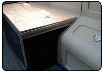
Position the bench seats to span the two side panels nearest the corner panels on either side of the camper/shelter. The back of the bench seat rests on the angled side of the panel.
