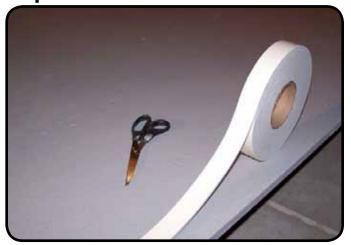
(Optional) Apply foam insulation tape (available at home improvement stores) to the floor where panels will sit. This helps prevent moisture and dust from collecting under the floor liner.
