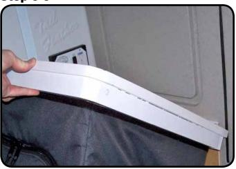
Unfold the cabinet and position the center shelf in the middle of the cabinet by fitting the shelf channel over the support rod. Lower the cabinet onto the cabinet brackets.
