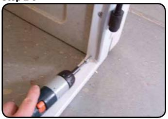
Insert a screw without washer into the hole at the bottom right hand corner of the door frame. This screw should line up with the slot in the end panel tab.
