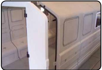
Align the door frame with the end panels. Push the door frame onto the panel tabs. (TIP: The center tab may not appear to line up, but it will pop into place with a firm push.)
