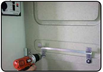
Attach the cabinet brackets to the side panel using the short 1/4" screws.
